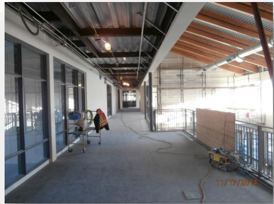
Second Floor Corridor
