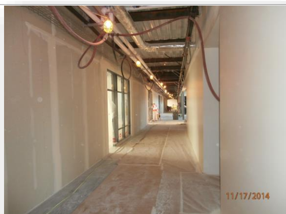
Second Floor Corridor
