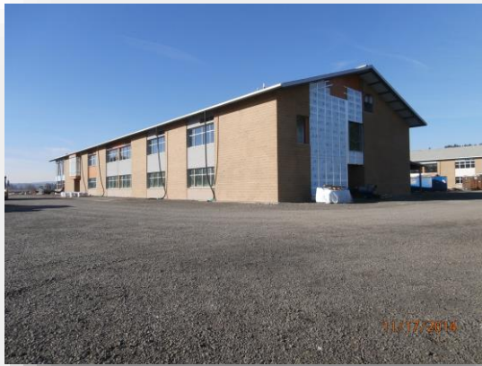
South Classroom Wing
