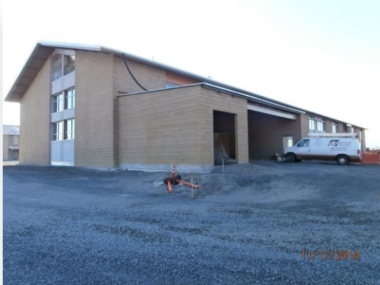
East end of North Classroom Wing
