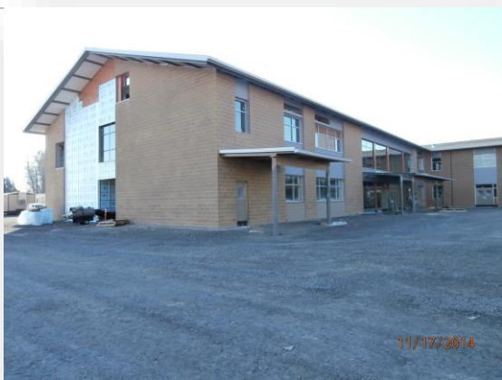
East end of South Classroom Wing
