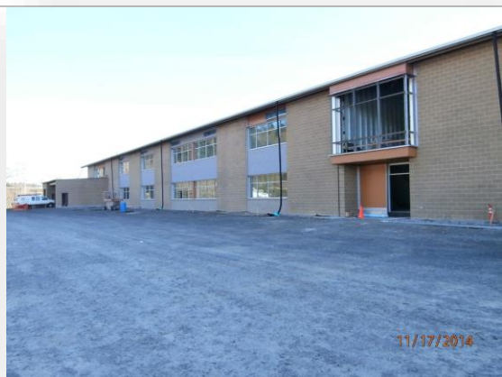
North side of North Classroom Wing
