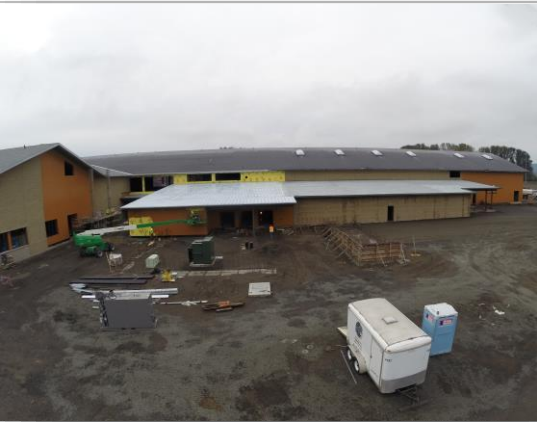
North side – Service entry, locker rooms
